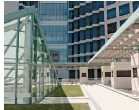
A balcony courtyard at the Simmons Cancer Center
